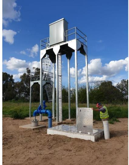
Figure 8 – Bunglegumbie No. 1 production bore site prior to construction of palisade fencing and surrounding concrete hard stands. All electrical infrastructure, contained within the grey switchboard atop the platform has been positioned at the Flood Planning Level, considered to be a 1% AEP flood with 500 mm of freeboard. The production bore and associated pipework is visible in the lower left of the photo, complete with stainless steel sealed bore head
