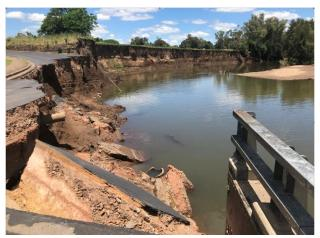
Photograph 5. Resultant damage to the reserve and approach to the southern end of the Duke of Wellington Bridge
