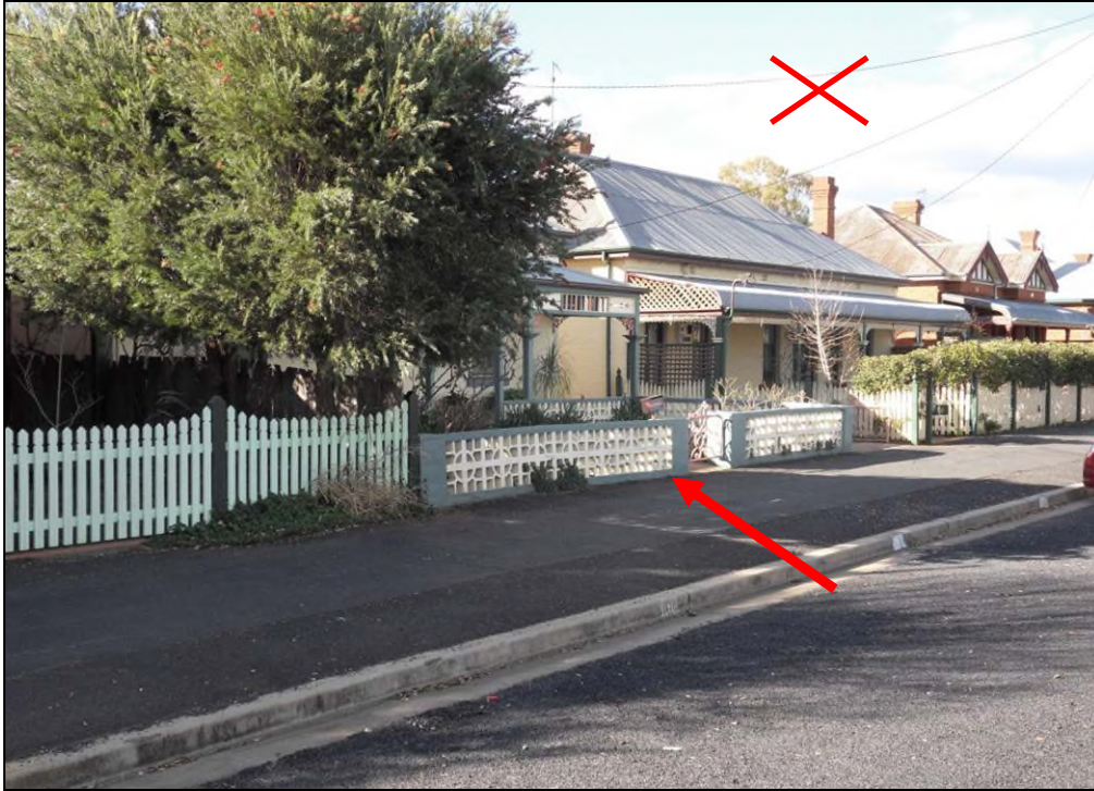
Fence height, style and materials are not compatible with adjoining fences.
