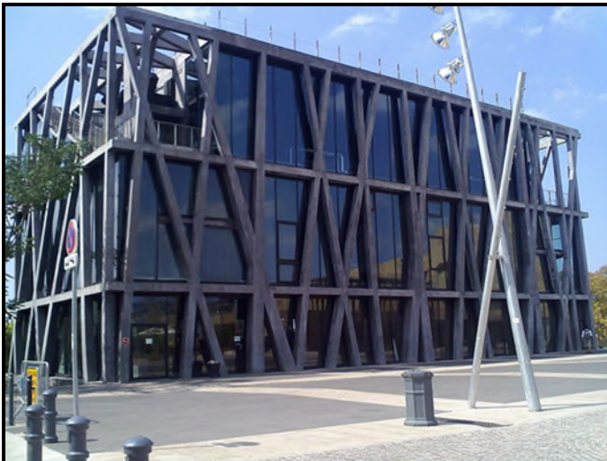
Photograph 2: This modern three-story building illustrates the architectural concept of expressed structure. The sloping columns and braces provide both the gravity and lateral support for the structure. The structure is cast-in-place concrete.
