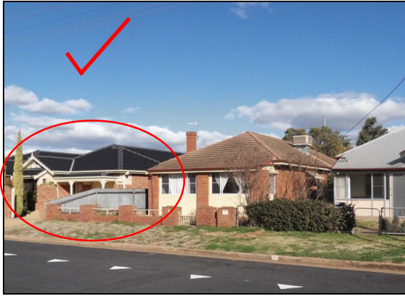
Infill dwelling that conforms to existing streetscape.
