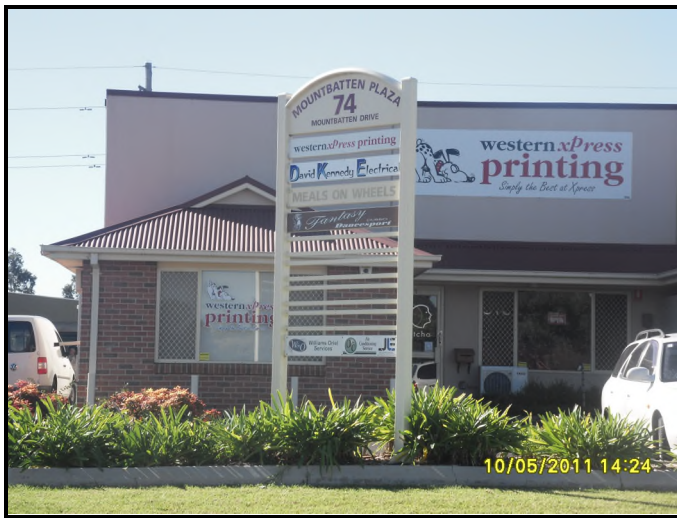
Photograph 5: The directory board sign provides all occupants with the opportunity to advertise their business and location. Behind, the fascia sign above the specific unit provides business identification.
