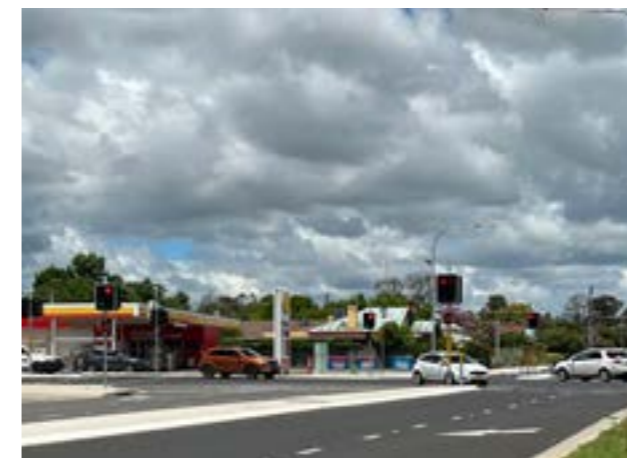
Cobra and Fitzroy Streets intersection Upgrade
