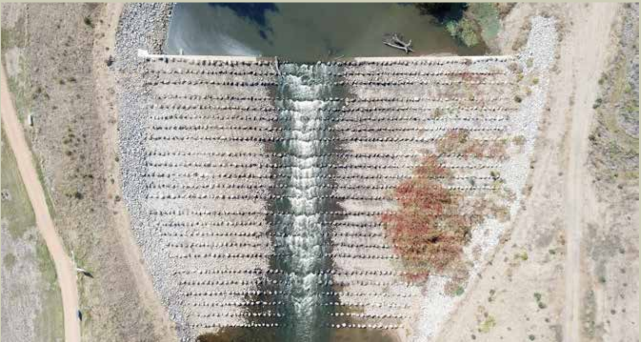
Upgraded South Dubbo Weir, including rock ramp and fishway.
