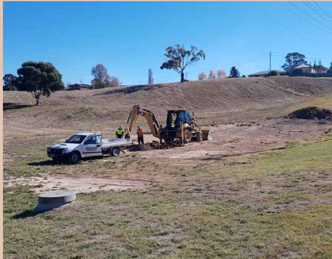
Investigating to determine the presence of Natural Occurring Asbestos in the Common, Oberon (Oberon Council).
