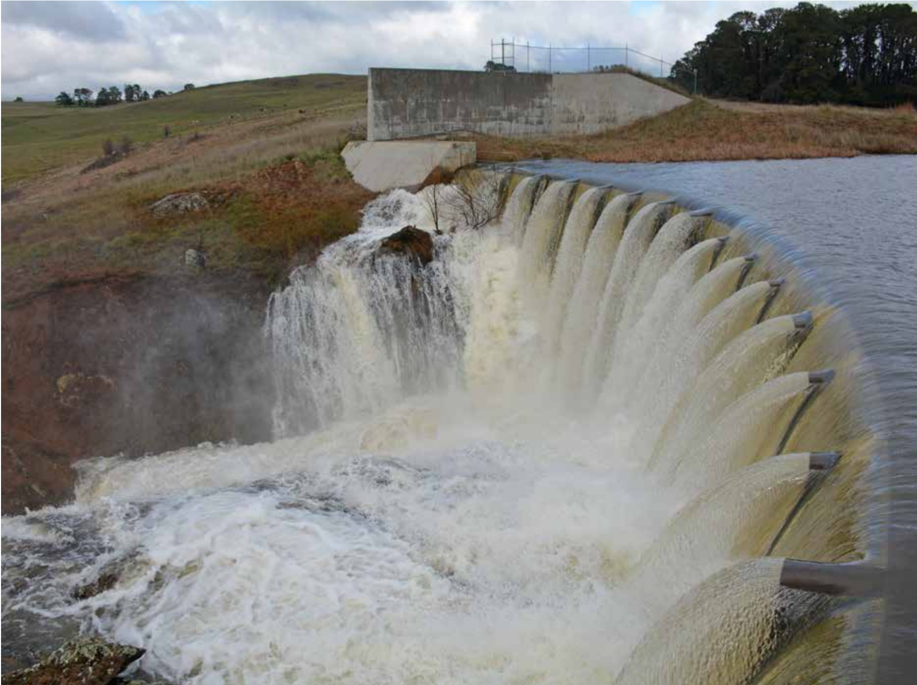
Spring Creek overflows, Orange LGA
