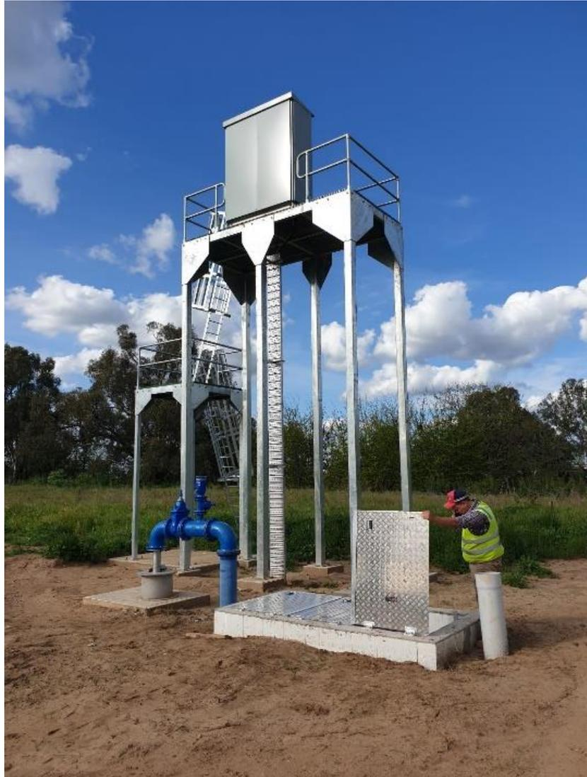
*Figure 8 – Bunglegumbie No. 1 production bore site prior to construction of palisade fencing and surrounding concrete hard stands. All electrical infrastructure, contained within the grey switchboard atop the platform has been positioned at the Flood Planning Level, considered to be a 1% AEP flood with 500 mm of freeboard. The production bore and associated pipework is visible in the lower left of the photo, complete with stainless steel sealed bore head*
