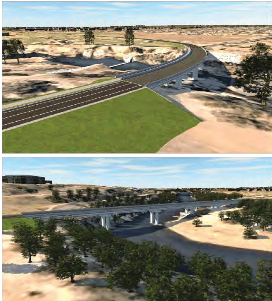
Figure E-1 Sample Images of proposed South Bridge – Top image is Option B (curved Bridge); Bottom image is Option A (straight Bridge)
