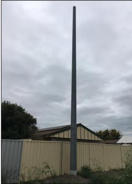
**Figure 2:** Existing sewer vent pipe along eastern boundary.
