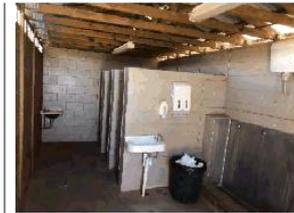
Image 4: Due to the age of most of these facilities – current BCA requirements for accessible (unisex) facilities and ambulant facilities, door widths, landings and graded paths to these blocks are not to code or evident.
