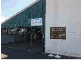
Image 4: Due to the age of this facility – several components (amenities, doorways, landings and general access would not be considered compliant current DDA and BCA requirements.
