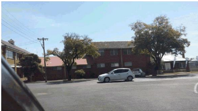
Plate 3: TAFE buildings in Fitzroy Street
