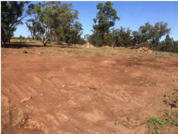
West across footprints of Stockpiles, D, E and F
