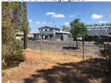
Image 8: Majority of fence line is Chainwire and is in a fair condition.
