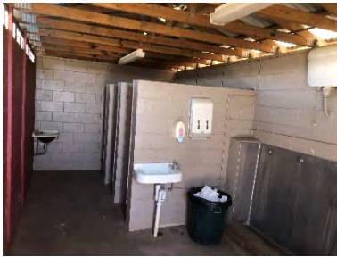
Image 4: Due to the age of most of these facilities – current BCA requirements for accessible (unisex) facilities and ambulant facilities, door widths, landings and graded paths to these blocks are not to code or evident.
