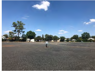
Image 8: Extensive paved (asphalt) area for showgrounds with minimal drainage and services connection.
