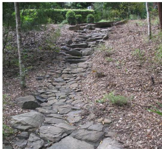
*Dividing plant groups by a drainage swale 'path'*
