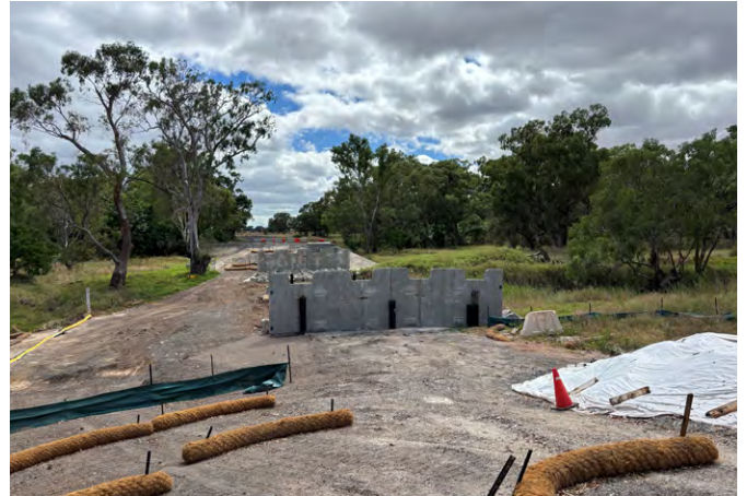
Construction of Comobella Bridge.
