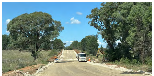
Ballimore Road reconstruction.
