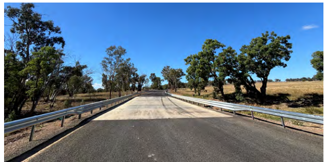
Burrendong Bridge No 1.
