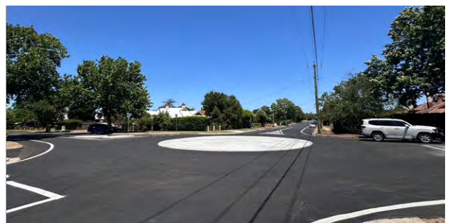
Tamworth and Darling Street roundabout.
