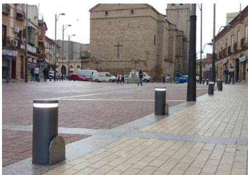
Telescopic bollards obstruct vehicles as needed. Toledo, Spain.
