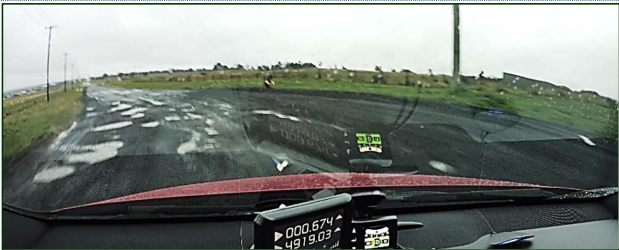
F8.3: Eastern section, northern turn, deep potholes and deep windrows of loose material on the outside of the curve.
