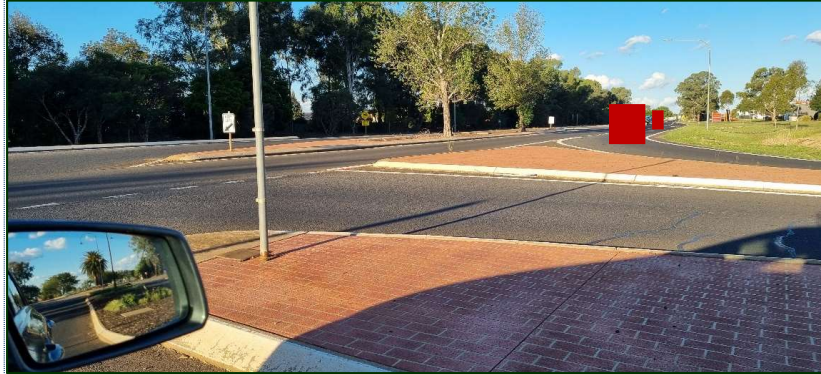
F7.2: Looking east, representation of sighting obscured by vehicles (represented by the red rectangles) turning left.
