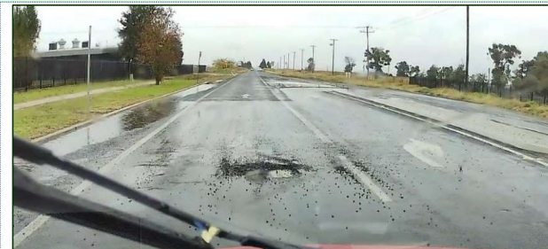
F5.4: Loose material, pothole, and water ponding.
