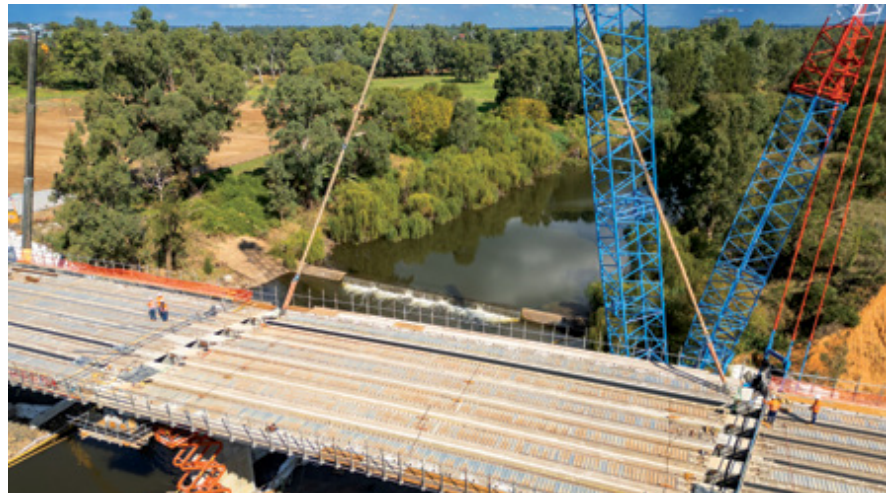
Final girder lift underway on the New Dubbo Bridge project
