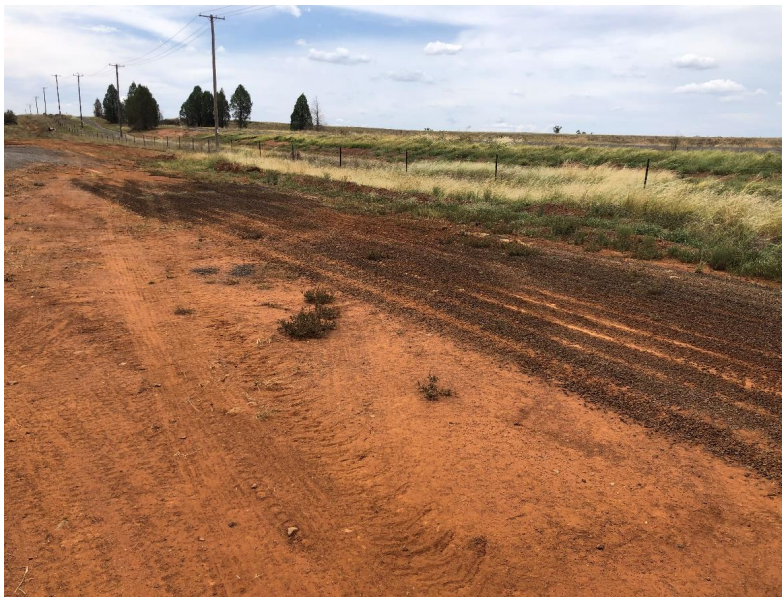
Figure 4.3: Remnants of bitumen covered roadbase material along eastern boundary.
