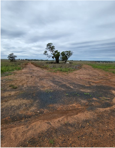
Figure 5-8: Stockpiled fill containing mixed road material, bluemetals and sand
