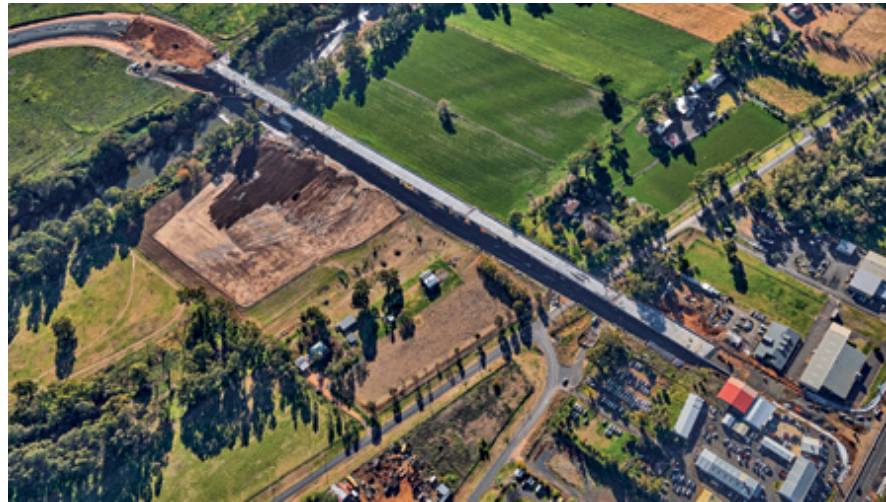
Figure 2. Aerial photo of the New Dubbo Bridge nearing completion
