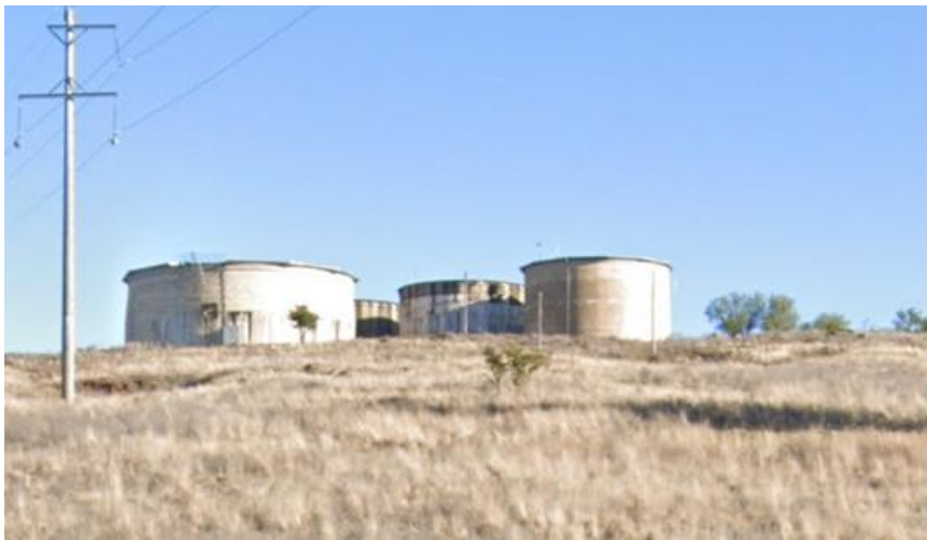
Picture 1. The two reservoirs in the forefront of the picture are in operation. The reservoir to the left has a capacity of 3.4 ML and the reservoir to the right has a capacity of 1.25 ML
