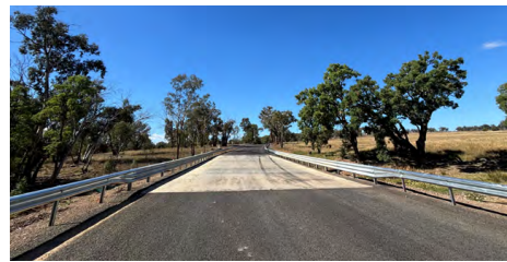
Burrendong Bridge No 1.
