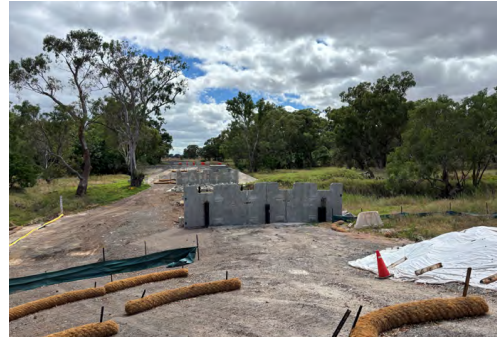
Construction of Comobella Bridge.
