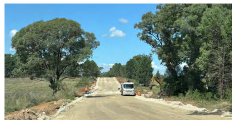
Ballimore Road reconstruction.
