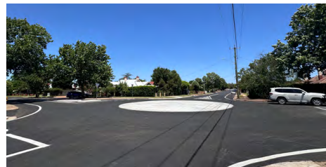
Tamworth and Darling Street roundabout.
