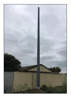
Figure 2: Existing sewer vent pipe along eastern boundary.
