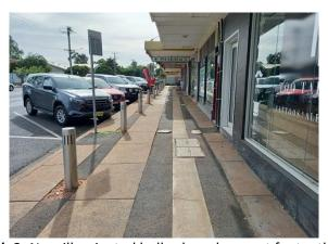
Photograph 3: New illuminated bollards and current footpath condition
