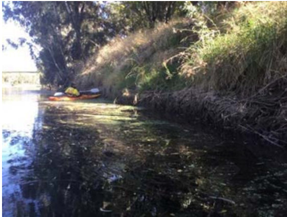
Figure A6.5 bank erosion
