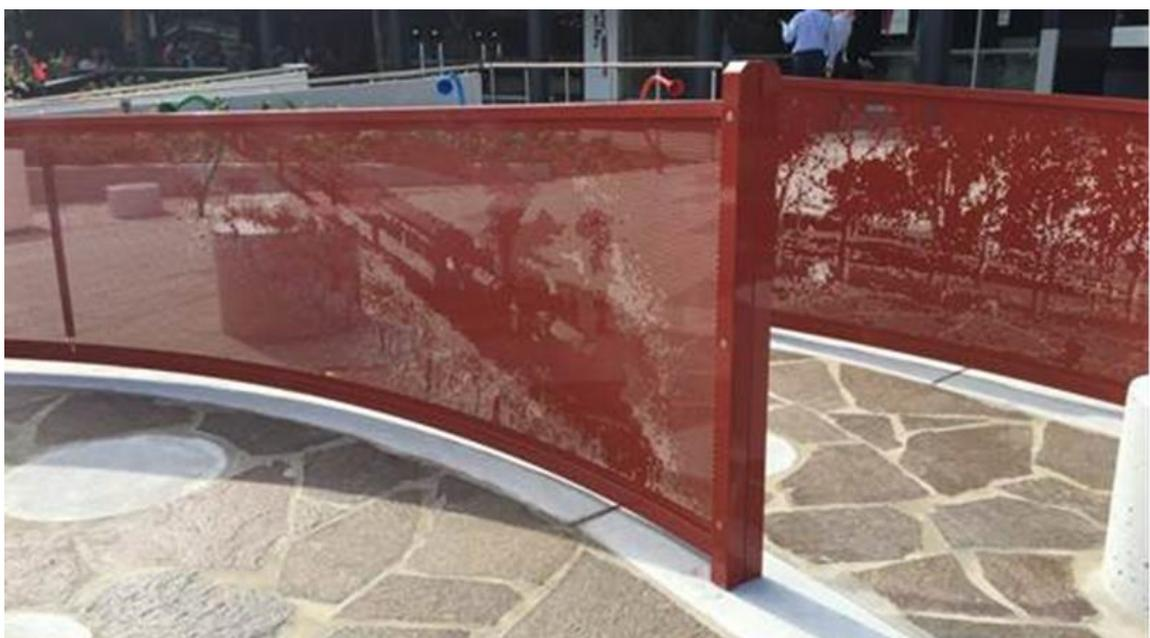
Figure 3 – printed perforated 3mm Aluminium fencing – dot matrix
