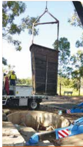
The GPT is emptied on a regular basis to ensure that it is always operating at optimal efficiency.
